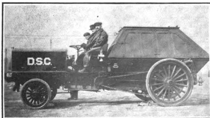
Convict-built truck with body in normal position—doors closed. Note drive-chain
